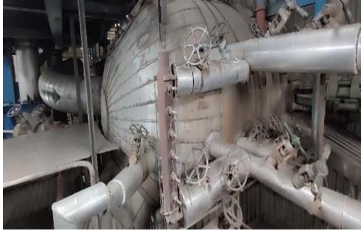
Gambar II.3.4.2 Steam Drum Boiler
