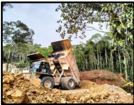
Gambar 2.12 Proses Penimbunan Material Waste
