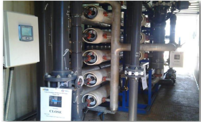
Gambar 1.8 Brackish Water Reverse Osmosis
