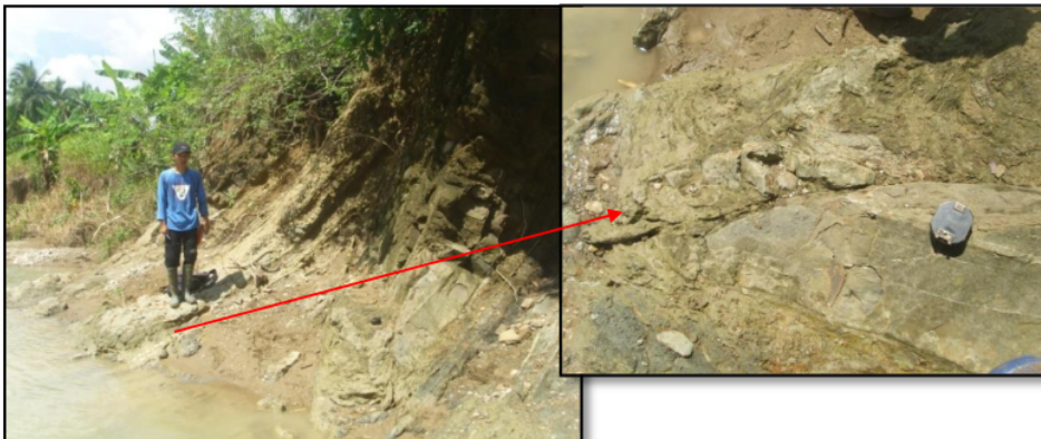
Figure 12. The appearance of Panimbo faults (Reverse Left Slip Fault (Rickard (1972))) in Kerek Formation in the Panimbo Village, Wonosegoro District, Boyolali Regency - Central Java
