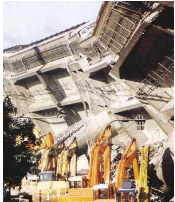
Collapse of Hanshin Expressway
