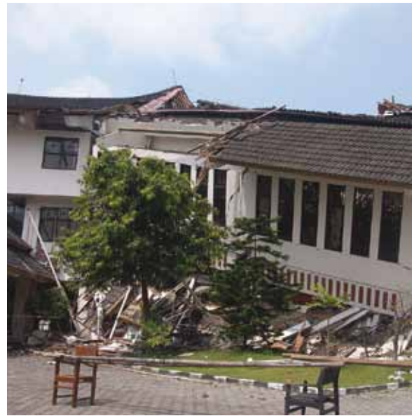
Damage of an engineered building caused by soft story, Yogyakarta 2006
