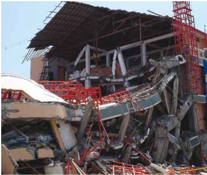
A four story engineered building damaged by earthquake in Banda Aceh, 2004
