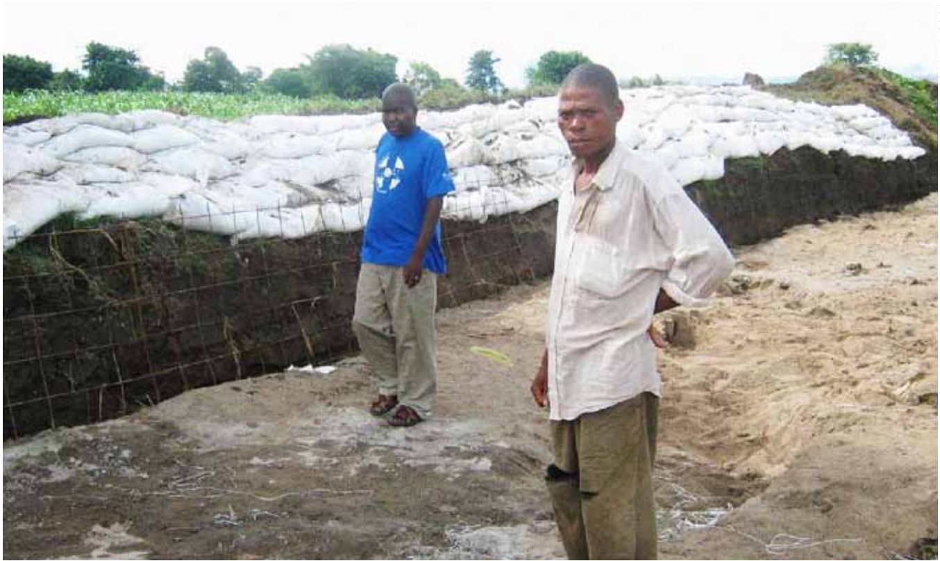
A GOAL engineer inspects the foundations of the planned gabion wire mesh reinforced concrete lining at Nyachilenda river
