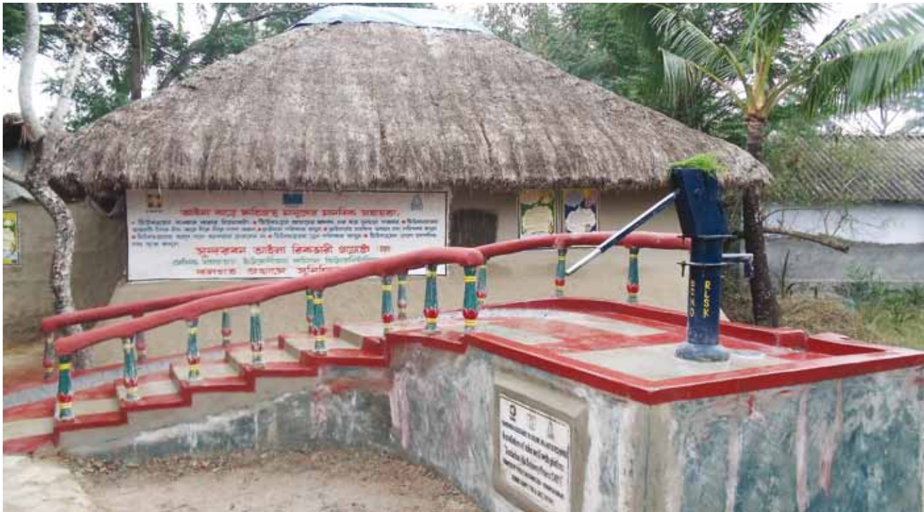
Raised handpump installed in Bidhan Colony Village; note the instructions on operation and hygiene promotion messages
