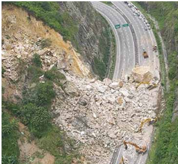
Rockfall along the main highway near Kuala Lumpur. Landslides on man-made slopes are the most common hazards for the Southeast Asia region
