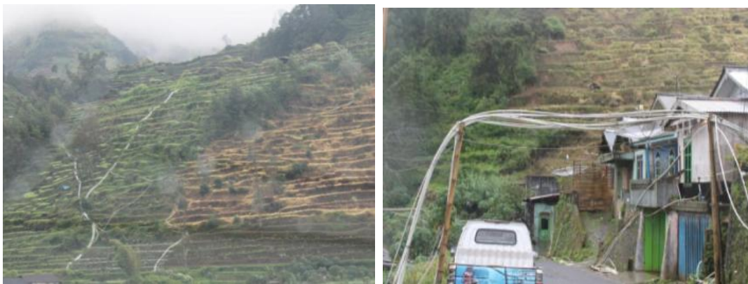
Fig. 2: PVC pipelines to distribute irrigation water from the downhill to the uphill
