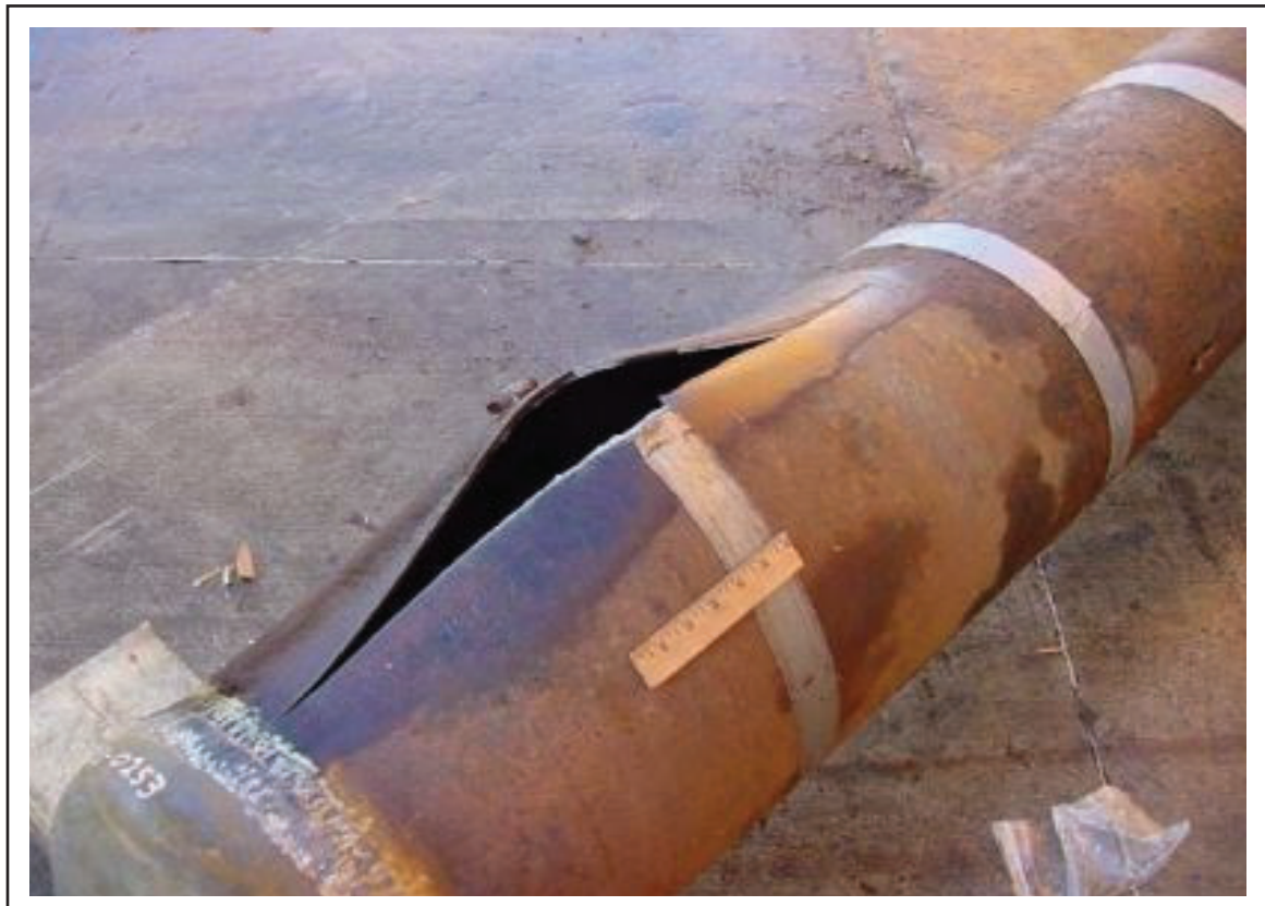
Figure 2 Casing when burst rating is exceeded.
