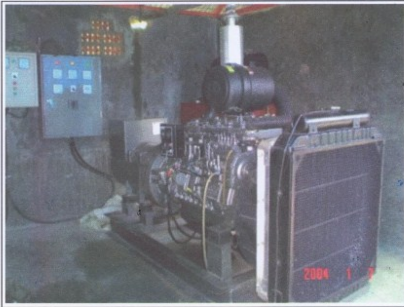
Gambar 7. : Genset Power Suply APTG
