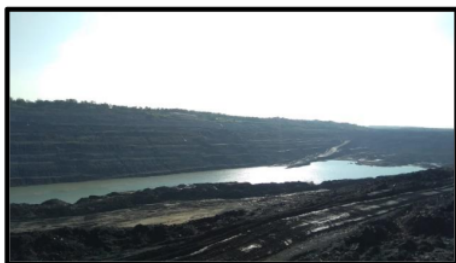
Gambar 4.2 Kodisi Lereng High wall
