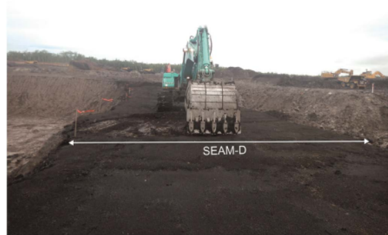
Figure 7. Correlation profile method in Seam-D assisted by units of excavators.
