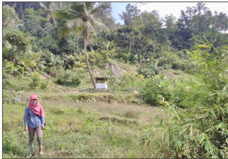
Figure 3. Landslide slope in Clapar village.
