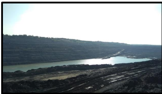
Gambar 4.2 Kodisi Lereng High wall
