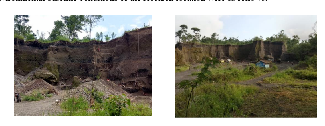
Figure 1. The condition of the living environment of the research location
