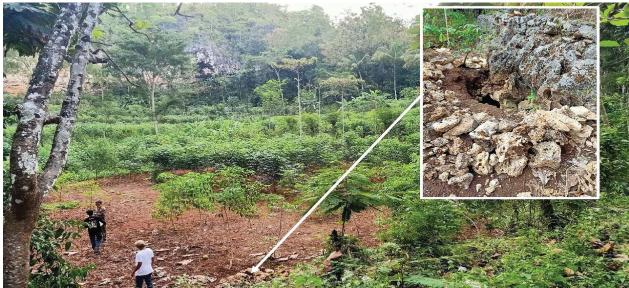
FIGURE 2. Location of the crack from local information. The area of the crack is on vast plain surrounded by cliff.
