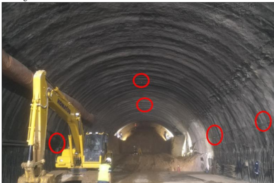
Figure 4. Prism-target position
