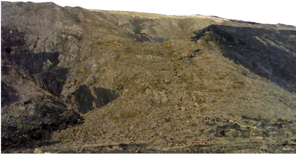
Figure 2 Low wall failure in the SIS pit of Tutupan coal mine
