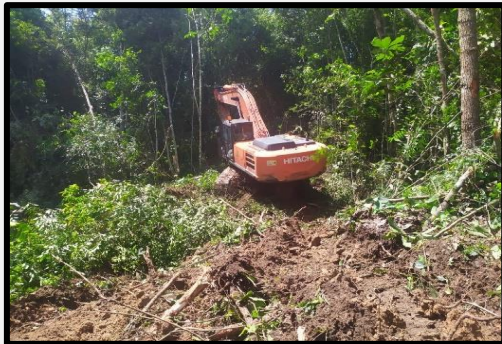
Gambar D.1 Land Clearing
