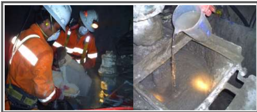
Gambar 8. Proses Pencampuran water cement ratio 0.35
