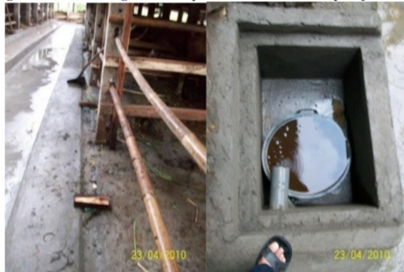
Figure 3. The hygienic communal fence that can divide urine and feces easily
