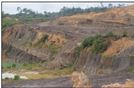
Fig. 2 Steep slope condition at the location
