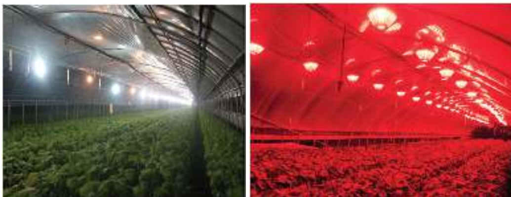
Fig. 6. Treatment of day length extension using by conventional incandescent (left) and red LED lighting device (right) in perilla at plastic house (Hong et al., 2012)
