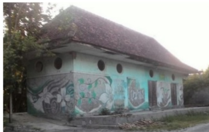
Figure 4 – Winongo Ex Train Station
