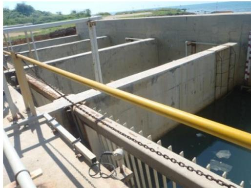
**Gambar 7. Sea Water Intake Kanal**
