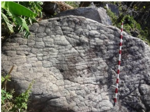
Fig. 14: Tortoise crack with planar flow appeared in agglomerate at Mt. Lawang
