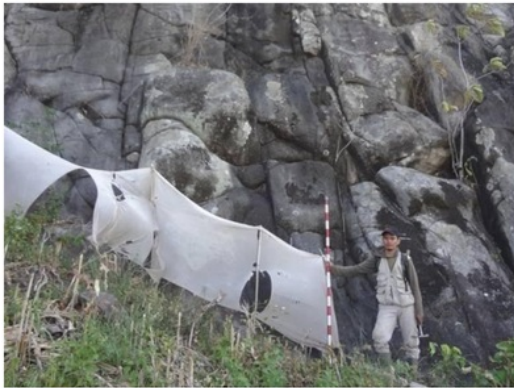
Fig. 12: Columnar joint structure at Mt. Lawang.
