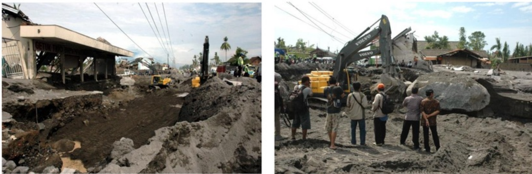
Fig. 9. Lahar of River Putih that has broken Yogyakarta – Magelang transportation line
