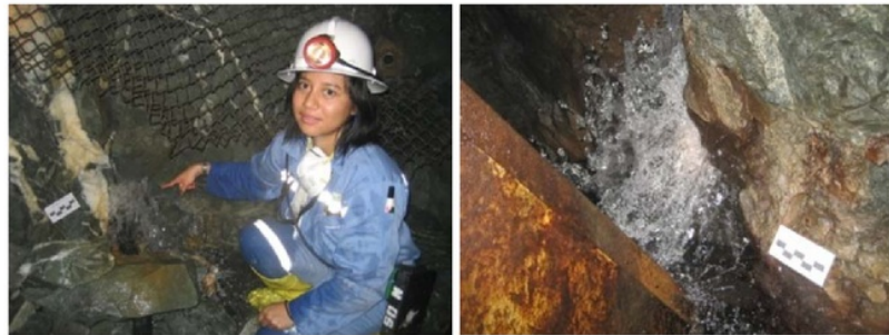
Figure 9 Groundwater inflows through fractures to the tunnel (see online version for colours)
