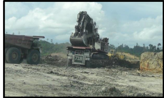
Gambar 4.1 Kondisi Loading Point
