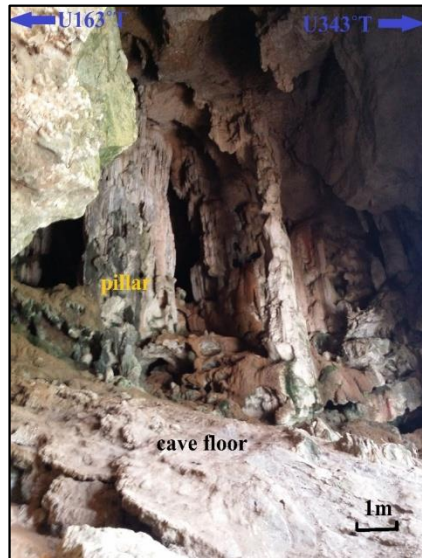
Figure 7: The presence of limestone pillars in the middle of cave act as support to prevent collapse of cave roof.
