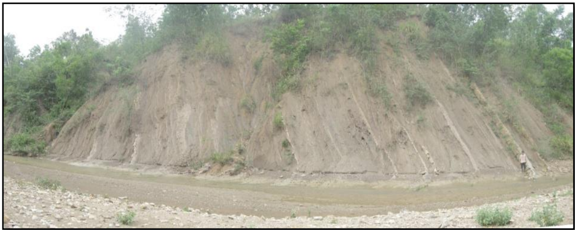
Figure 3. intercalation between sandstone calcareous mudstone which is dominated by mudstone, kerek Formation, on the Village Benge, District Wonosegoro, Boyolali Regency - Central Java.
